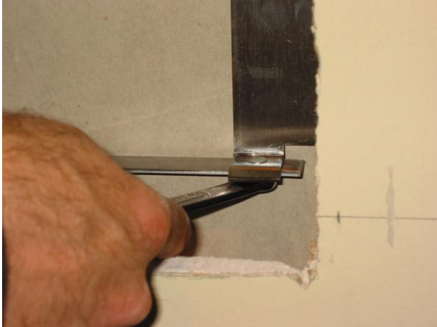
13. Tighten cross brace nuts using a 7/16" open end wrench.
