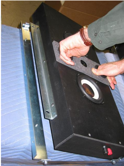
9. Separate the loudspeaker from the mounting bracket.
