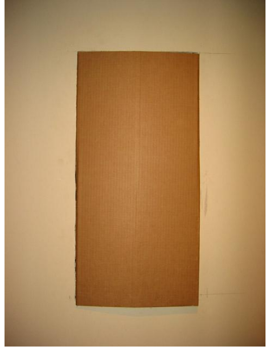
14. In pre-construction installations, the template may be reversed with the cardboard flaps in the wall, defining the bay as reserved.
