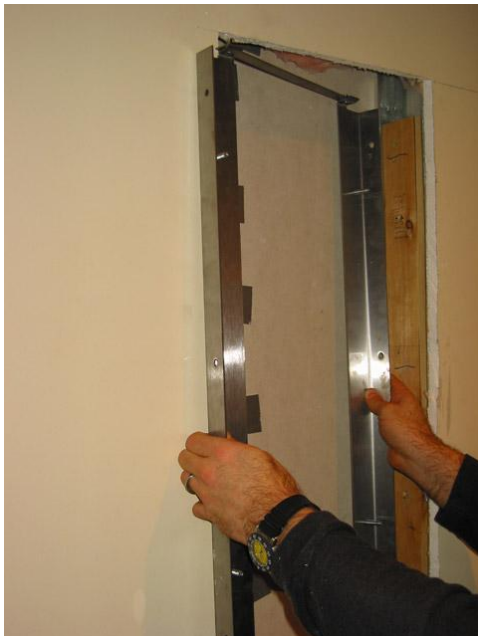
11. Place the bracket assembly in cutout, locating the bracket over the predrilled pilot holes.
